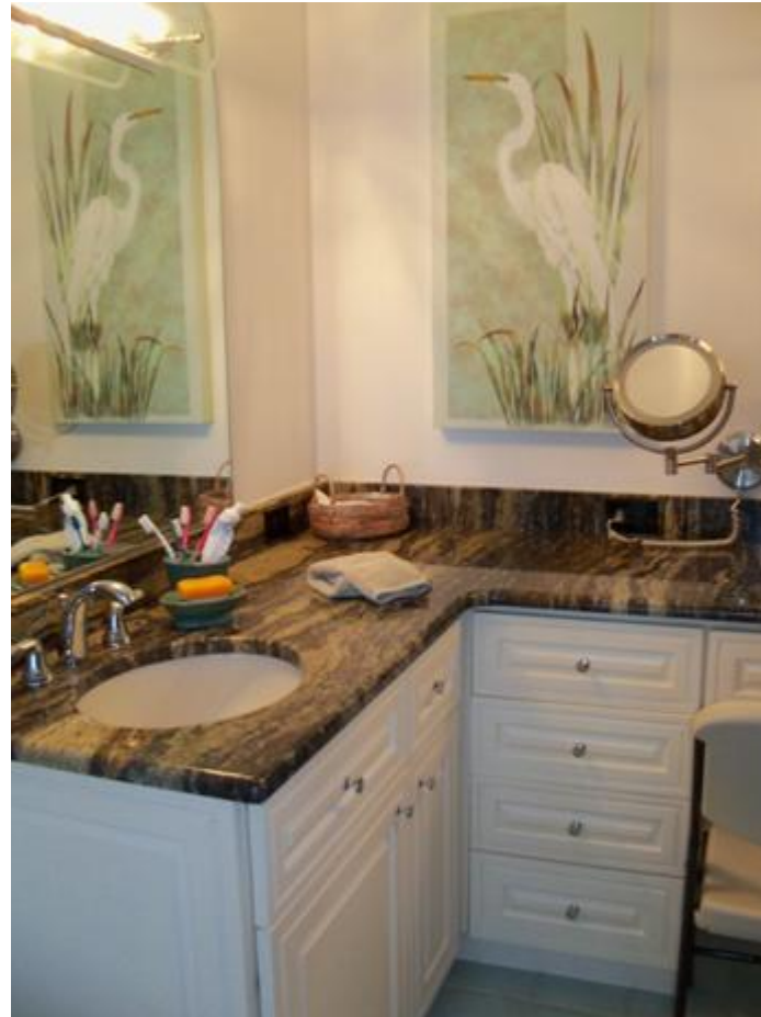
Uba Tuba granite countertop and backsplash installation in bath I
