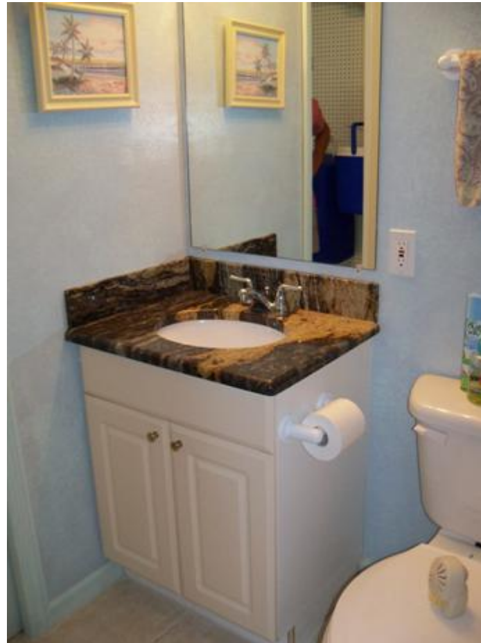
Uba Tuba granite countertop and backsplash installation in bath 2
