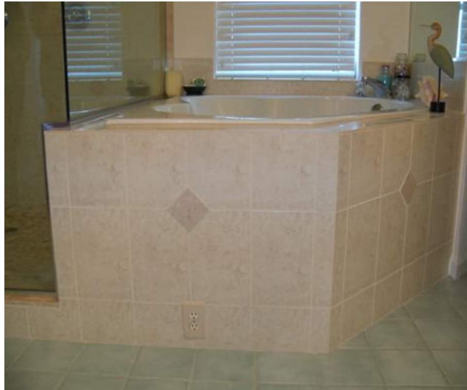
Tub wall tile installation
