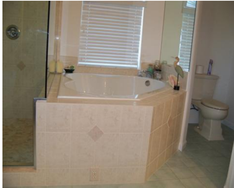
Tub Surround and backsplash tile installation
